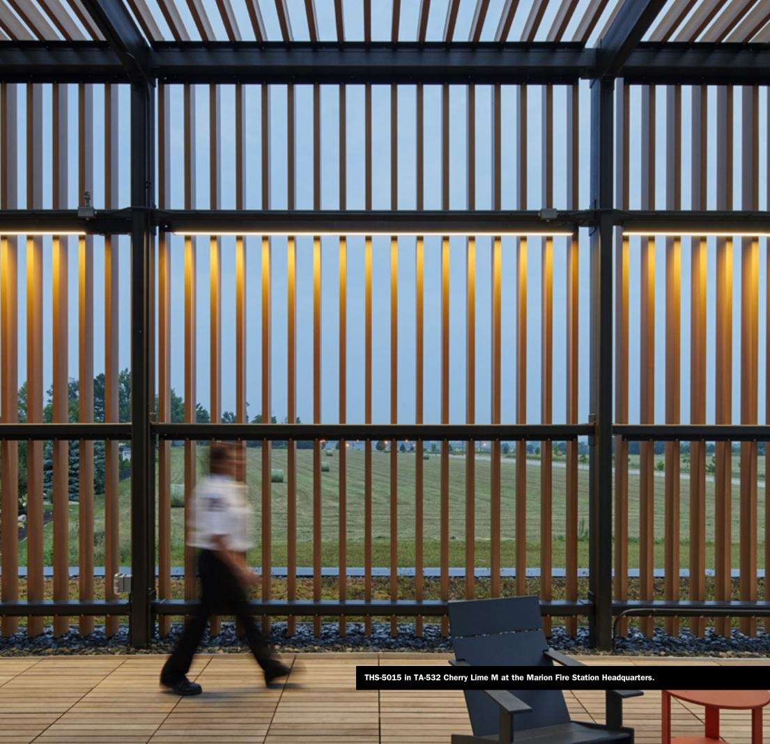
Battens are wrapped in an extremely durable non-PVC film. These films replicate real wood veneers with an astounding realism, indistinguishable from real wood but with a consistency and durability beyond actual timber.
