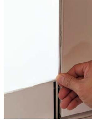
**STEP 3:** Using a finger, slide it across all four sides, pushing in the remaining gasket.
